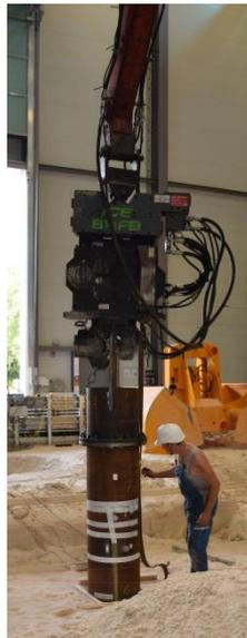
**Figure 16: Installation of Pile 2 with vibratory technology. Test campaign set-up by Fraunhofer IWES at the test centre for support structure in Hannover (Testzentrum Tragstrukturen Hannover, TTH), 2015.**
