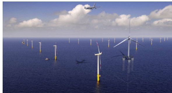
FIGURE 4.47 “Triple Spar” reference platform supporting the 10 MW INNWIND.EU wind turbine
