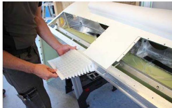
FIGURE 4.17 The flaps are manufactured in sections of 25 cm. Therefore 8 flaps are mounted side by side to constitute a complete 2 m long flap section.
