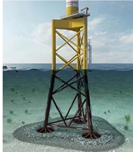
Figure 4.1-1: Jacket with bucket
