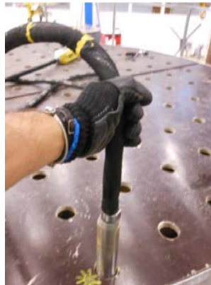
Figure 4.1-10: Vibration starts inserting the rod vibrator in the hole marked in yellow
