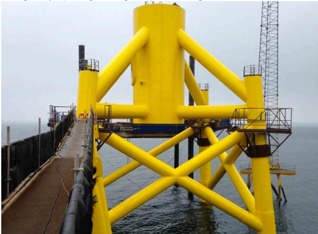
**Figure 6.1-5: Simple strut model with external platform to be placed on top of the TP chords [Fife Jacket]**
