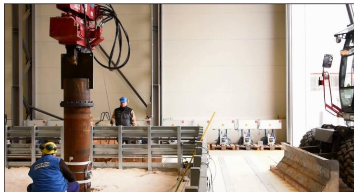
Figure 4.2-17 – Pile 1 at the end of the installation.
