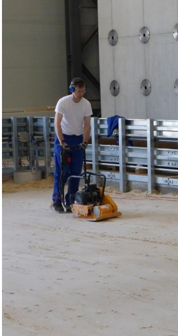
Figure 4.2-4 – Sand compaction of subsequent layers by using direction plate compactors.
