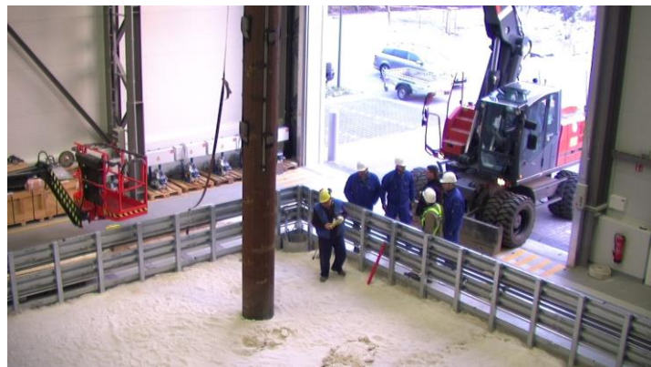
Figure 4.2-16 – Pile 1 at the beginning of the installation.
